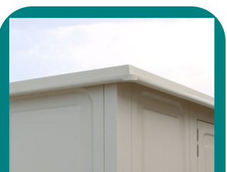
Roof Overhang in front 200mm
